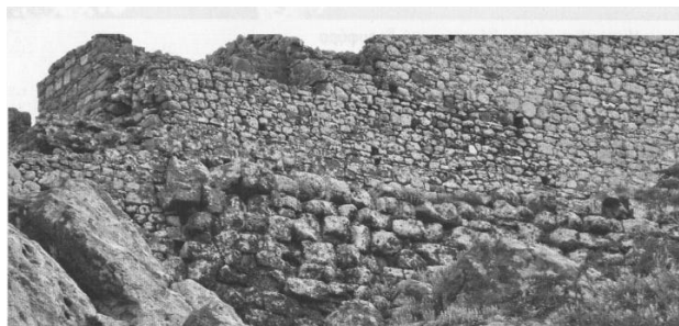
Venetian walls built on top of cyclopean walls on the North side of the Castle
