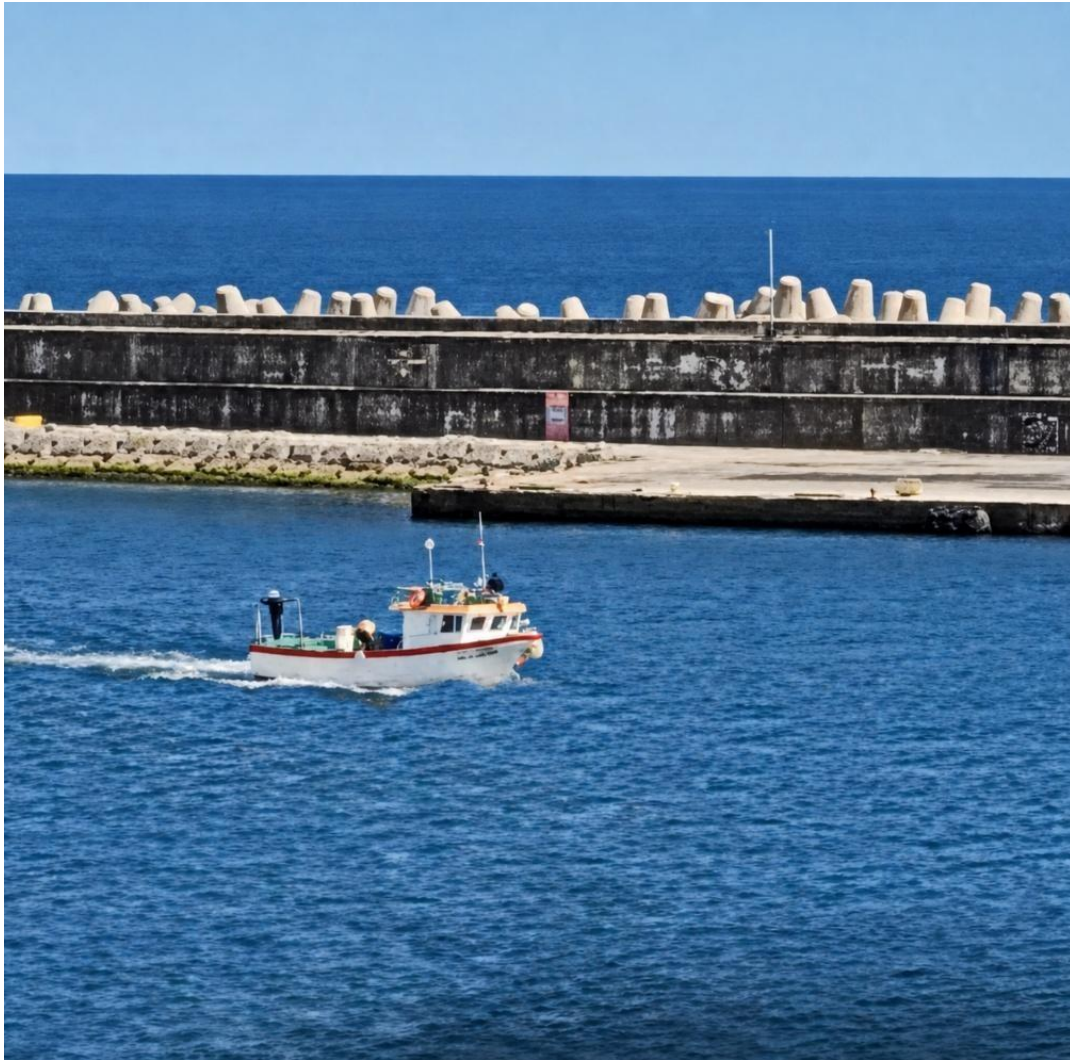
Ponta Delgada, 12-metre Protective Wall
